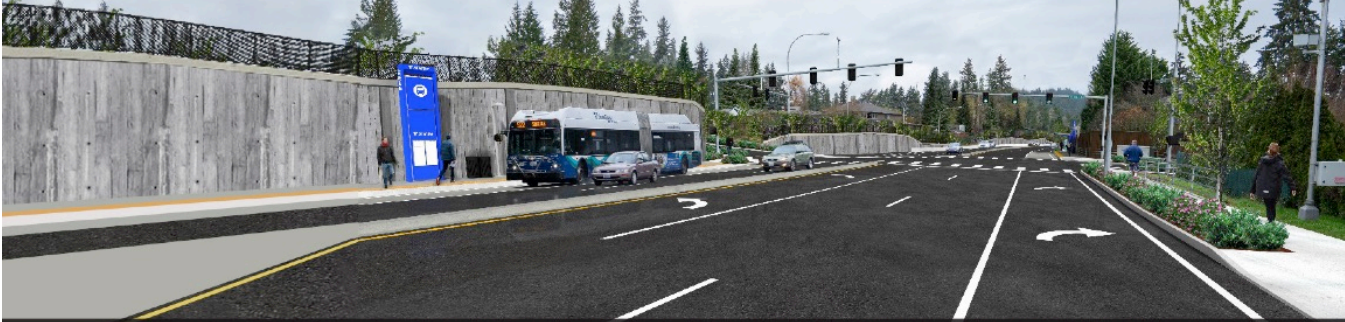
Stride S3 Wall and Black Chain Link Fence Do Not Provide Noise Mitigation or Landscape
